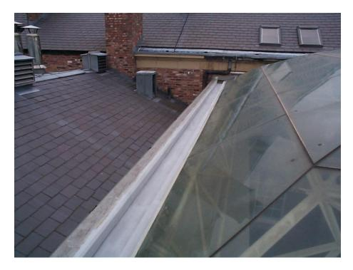
In this article prepared for RCI Magazine, Mark Bruchez, Technical Director at roof waterproofing specialists KEMPER SYSTEM, argues that failed guttering can usually be repaired rather than replaced - and that the result is likely to outlast alternative replacement options.
