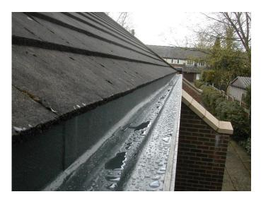
Deterioration of the original linings over time, due to differential movement and expansion, leads to failure resulting in leaks which can affect both the external wall and the cavity itself resulting in structural damage and dampness to the internal wall.
