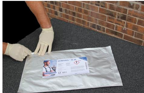
Use the side of your hand to evenly distribute the material within the aluminium bag. Tear open the bag with the help of the tear aid.
