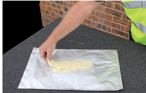
Carefully clean the dry surface to be patched, e.g. bitumen or PVC roof sheeting. Take out and put on gloves.
