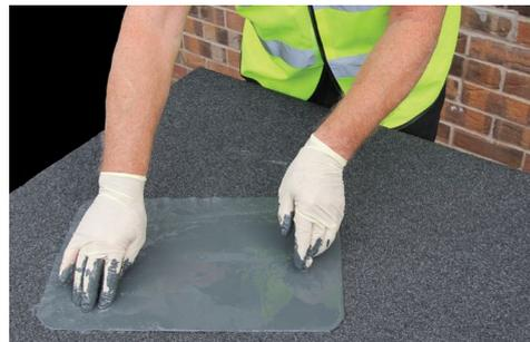
Position the aluminium bag over the area to be repaired. Hold the Roofpatch tight with one hand and carefully pull out of the aluminium bag and apply over the damaged area. Smooth the Roofpatch with your hands to remove any air bubbles or creases, and to ensure good contact with the roof substrate. Safely dispose of the gloves and aluminium bag. That's it. The surface is rainproof in around 60 minutes.
