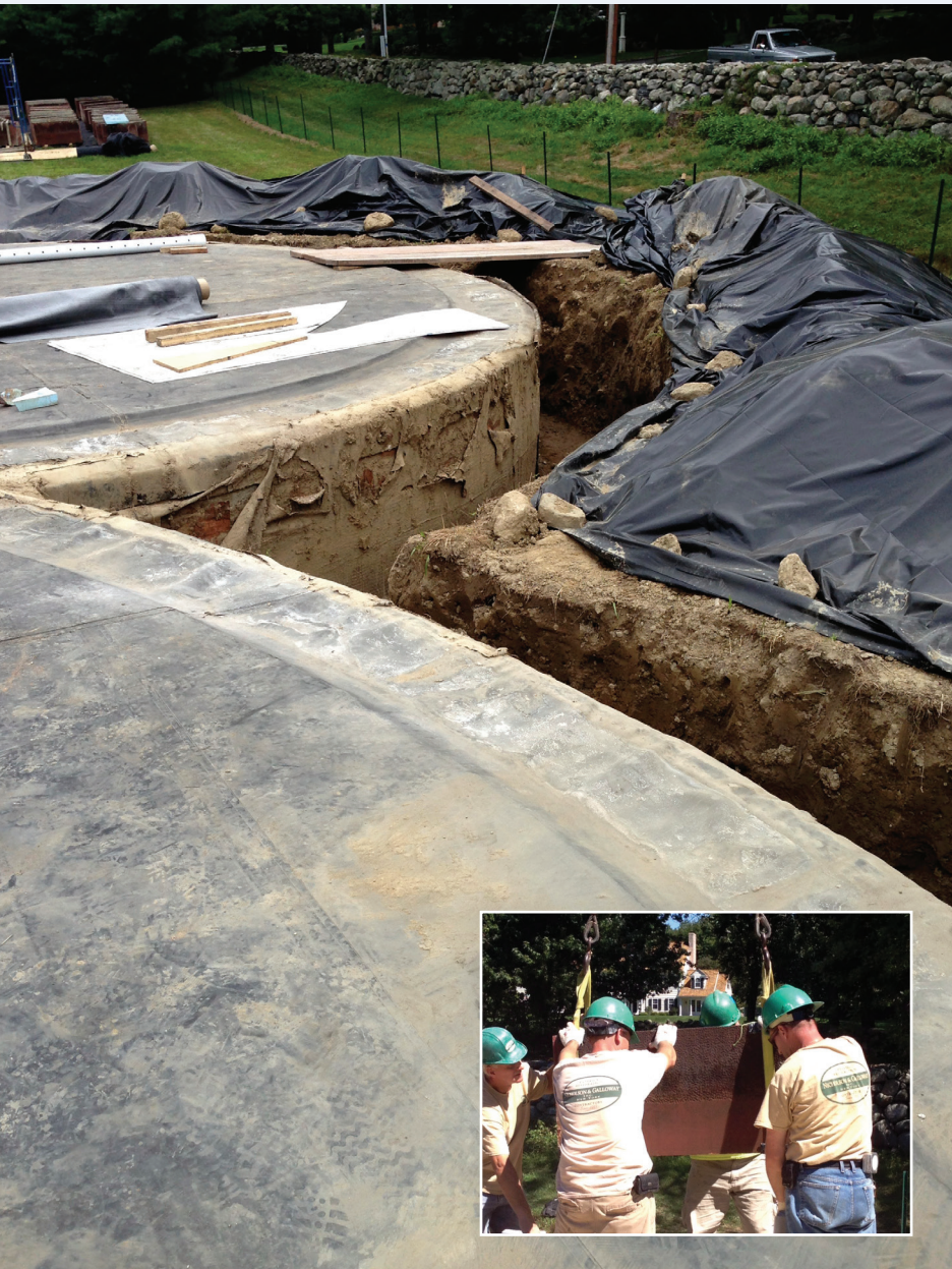
Heavy lifting - The project included removal of over 200 cubic yards of earth berm around the gallery and moving 54 Redstone copings by crane before roof work could get underway.
