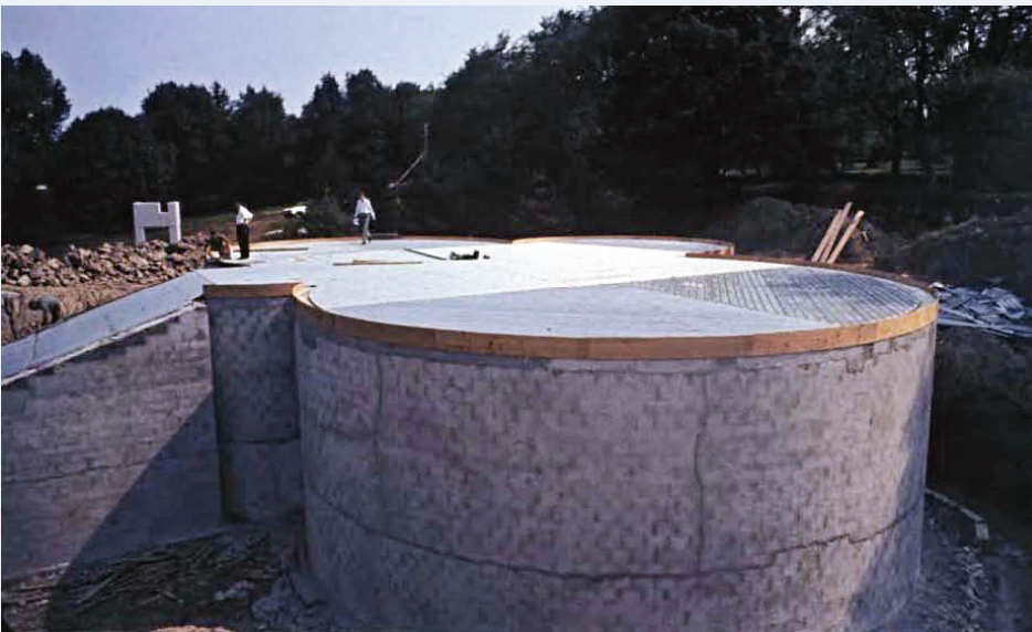
Construction (1965) - The 20 ft. high walls of the gallery were originally waterproofed in 1965 with a bituminous coating.
