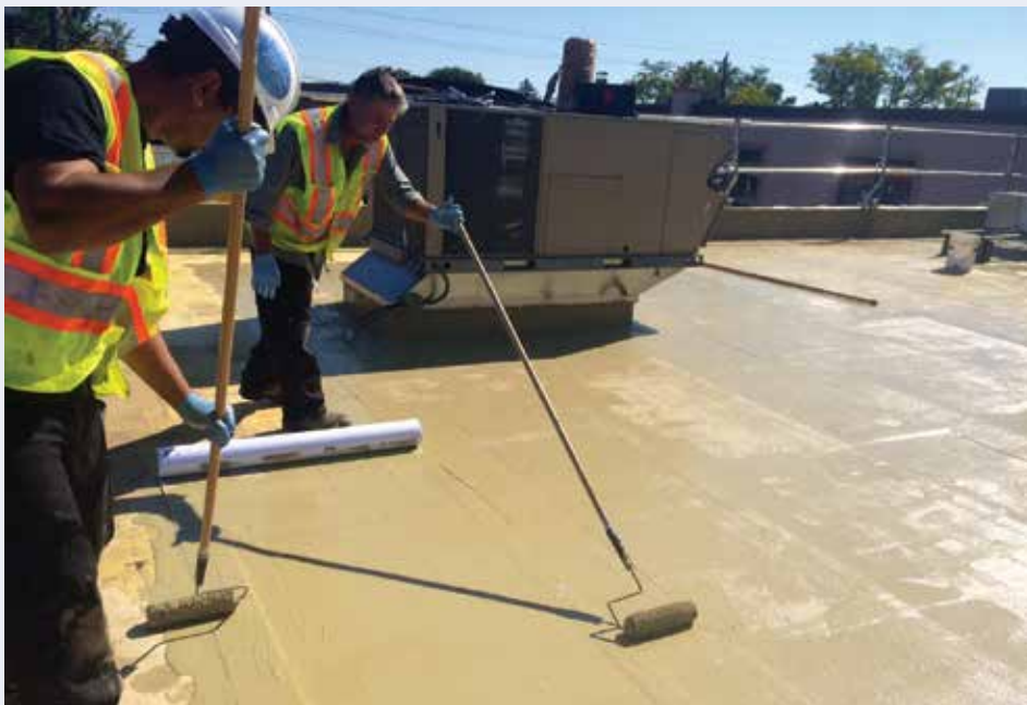
Shell Oil (above) In 2014, KEMPEROL® 2K-PUR system proved effective for reroofing Shell gas stations / convenience stores at pilot locations in Ontario. Hunter worked with the Shell facility manager to scope out the project, define specifications and identify certified applicators. “Odor-free, health and safety were important considerations,” Hunter says. Contractor: Flynn Canada Ltd. (Mississauga)
