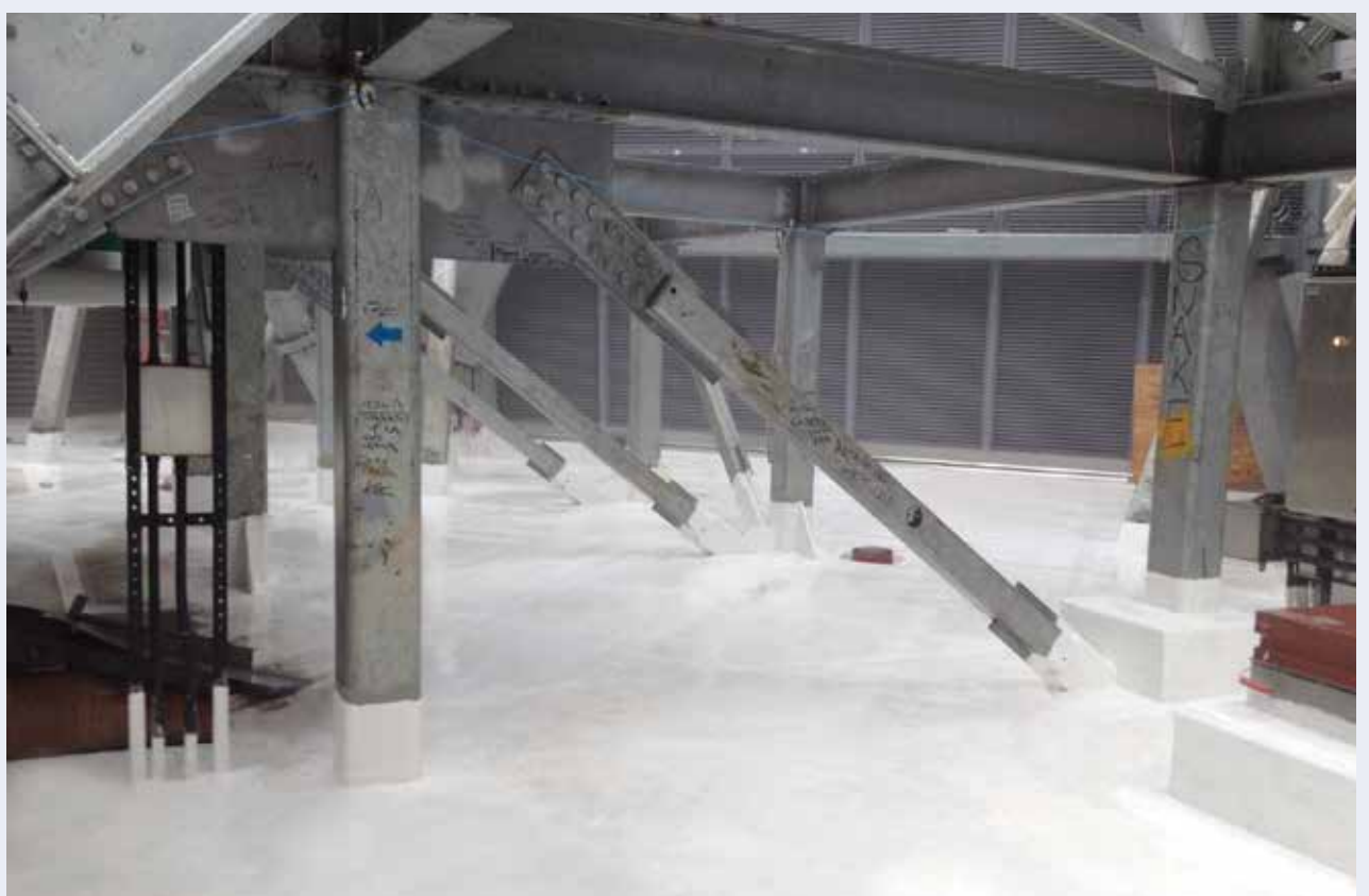
What appears to be a simple white coating is actually the top layer of the Kemper System. The KEMPEROL® membrane is fleece-reinforced and forms a seamless surface that is unaffected by standing water, snow or ice. It also resists chemicals and corrosives, and UV light.
