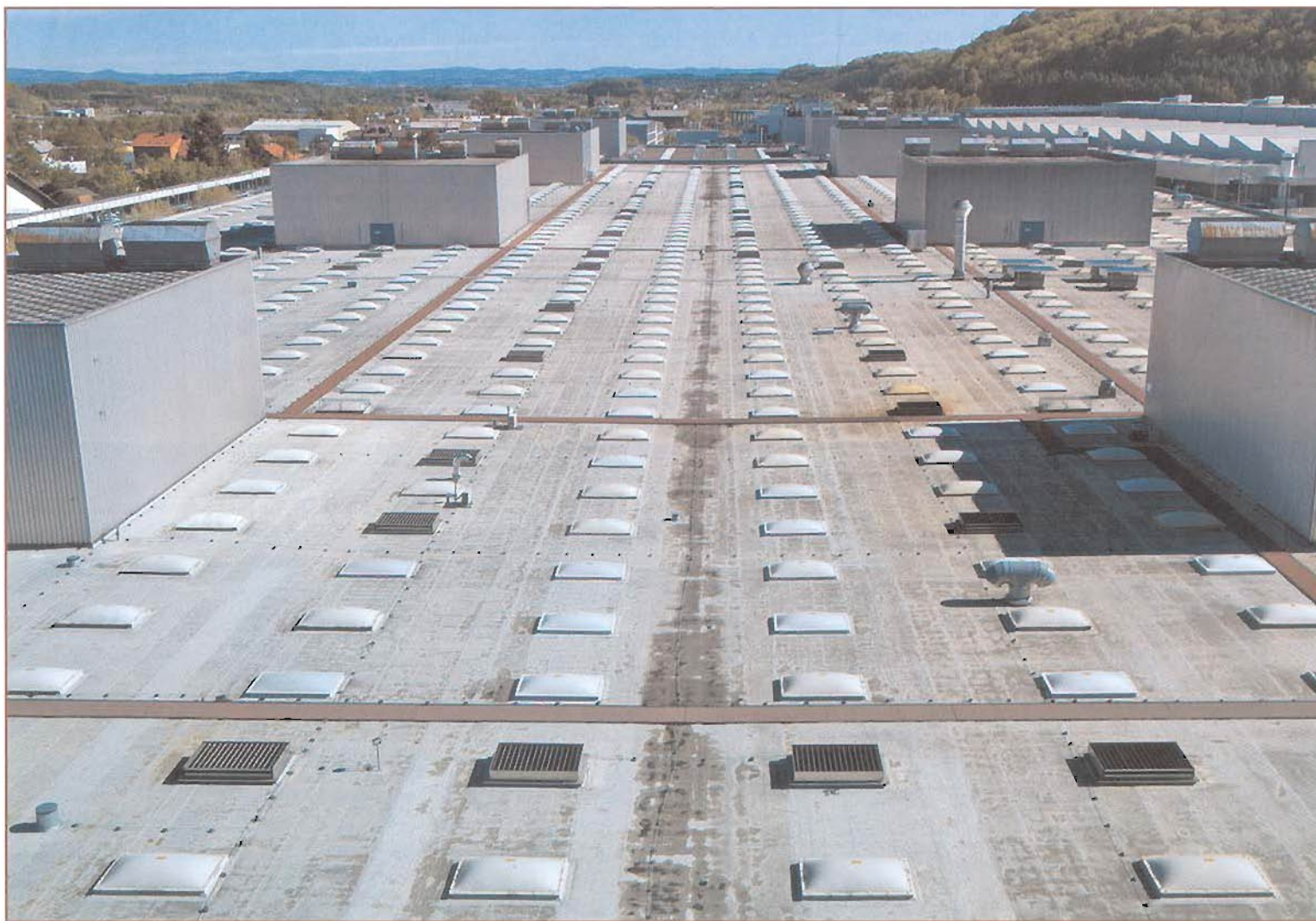
Some 646,000 square feet of liquid waterproofing have been laid over the various roof components on the BMW plant roof in Steyr, Austria, over the last 15 years.
