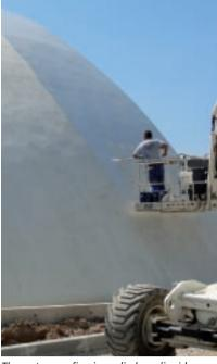
The waterproofing is applied as a liquid.
