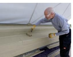
KEMPEROL® Waterproofing only came into contact with the special plastic fabric at the junction points, which were waterproofed separately. Application: The first layer of KEMPEROL® is applied, a reinforcing fleece is then embedded within this base coat, a second layer of KEMPEROL® is immediately applied as the top coat to fully saturate the wet fleece.
