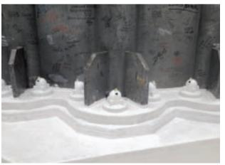
What appears to be a simple white coating is actually the top layer of the KEMPER SYSTEM. The KEMPEROL® membrane is fleece-reinforced and forms a seamless surface that is unaffected by standing water, snow or ice. It also resists chemicals and corrosives, and UV light. Huge bolts at the base of the spire were among hundreds of exposed roof details also protected with the KEMPEROL® waterproofing system
