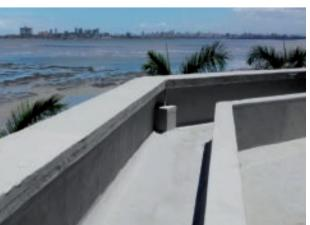
The roof above the server rooms was applied with KEMPEROL $^{\circ}$ . It protects the concrete structure and provides a barrier against salt water.
