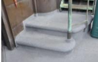
The observation deck of the Hamburg Michel was effectively waterproofed using KEMPEROL® and given hard-wearing-coating using KEMPERDUR®. Round shapes and many complex details-ideal for the application of liquid applied waterproofing
