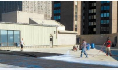
recreational surface were tested for compatibility. An acrylic adhesive is spray applied to the KEMPEROL® membrane to adhere the first of multiple layers of the sports surfacing.
