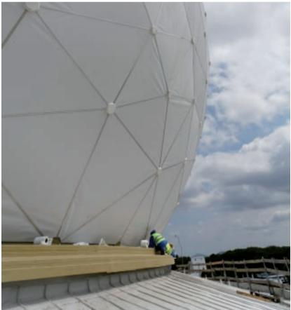
The concrete base was waterproofed using KEMPEROL® 2K-PUR.
