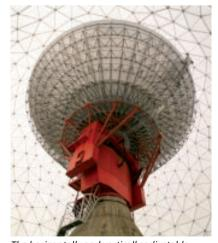
The horizontally and vertically adjustable parabolic reflector inside the dome measures 34 metres in diameter and weighs 240 tons.
